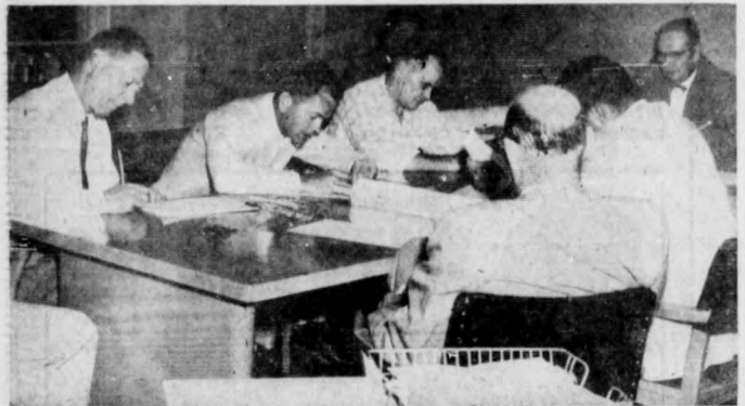
FIRST JOB CONFERENCE — Contractors for million-dollar addition to Plymouth-Whitmarsh High School meet May 22 to schedule work on project, climaxing long months of planning. Workmen moved on site May 24, erecting shack to house equipment, ready to begin construction.
