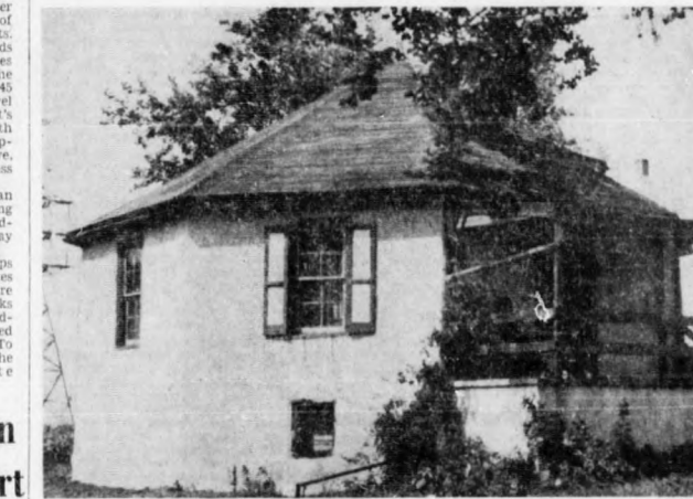
ERECTED IN 1818, the building above figured in the early educational and religious history of the community...
