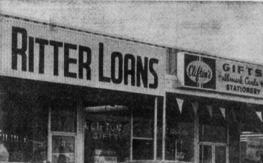
PROGRESS — Ritter Finance Co., formerly of Conshohocken, occupies one of the new offices in Plymouth Square Shopping Center. Largest unit is the A & P Supermarket. Additional stores are under construction, also a bowling alley, and, separated from the main center, the First Pennsylvania Banking and Trust Co. is raising a three-story brick dwelling on the site where it will open a branch in near future.
