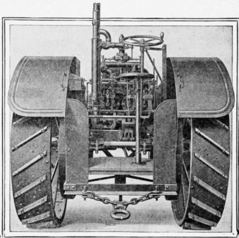
The convenience and comfort of the operator have been considered in the design of the International. Note the spring mounted seat and platform
