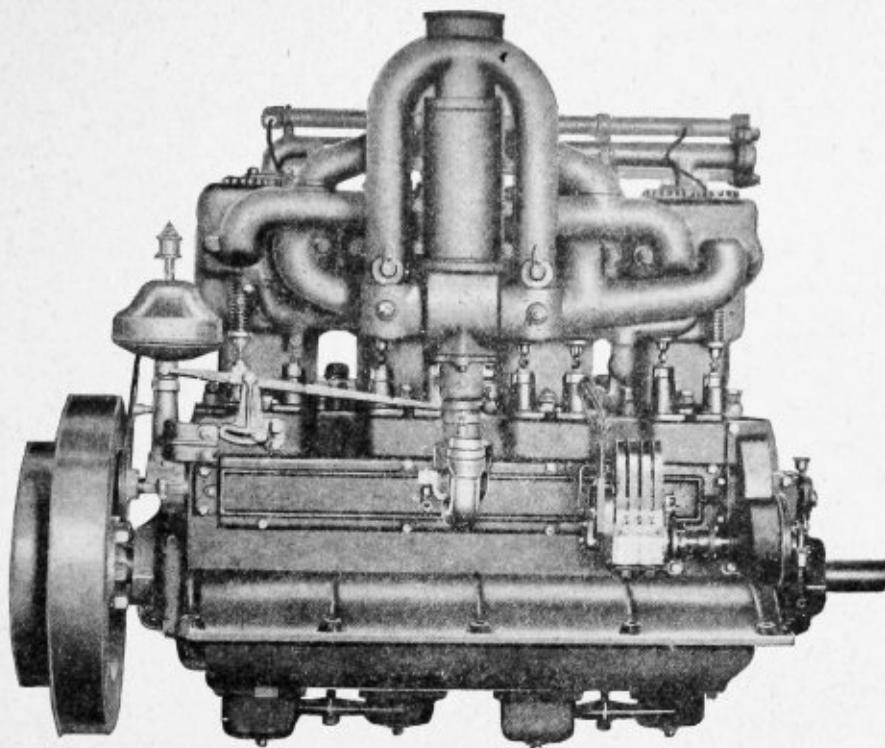
7 1/4 x 9, Four-cylinder Twin City Oil Engine, Valve Side
