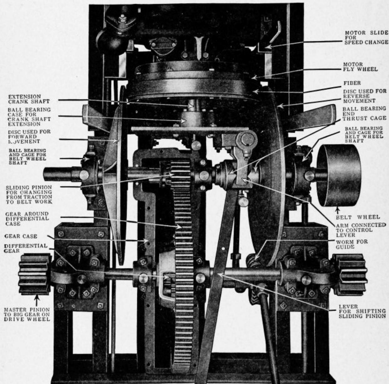
NOTE—THE FORWARD, REVERSE AND STOPPING MOTION IS ACCOMPLISHED BY THE SLIDING MOVEMENT OF THE BELT WHEEL SHAFT. THE DIFFERENT FORWARD AND REVERSE SPEEDS ARE ACCOMPLISHED BY SLIDING THE MOTOR BACK AND FORTH WHICH IS DONE BY A LEVER IN THE CAB.
