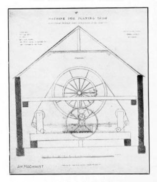
Although dated 78 years ahead of the hand planer shown on page 2 this planing machine, invented by Nicholas Forq, a French clock maker, is a considerable number of steps in advance as regards principle of design. Unfortunately the illustration lacks the carriage carrying the planing tool. The machine was used for planing the pump barrels used in the Marly waterworks to supply the fountains at Versailles.
