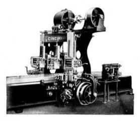
Can you imagine a greater contrast than is evidenced by these two machines; the crude model at the left and this last word in modern planer construction—the Cincinnati Electric Variable Speed Planer?
