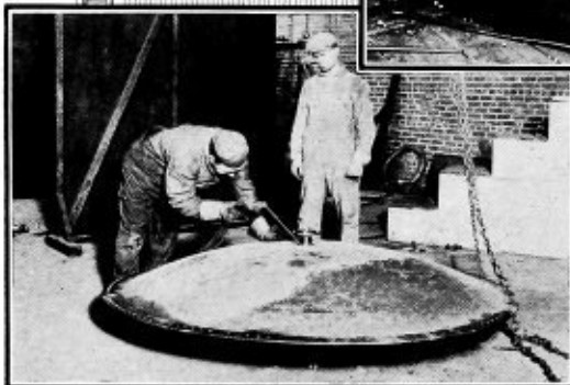
Application of Metal Electrode welding in the manufacture of Tanks.
