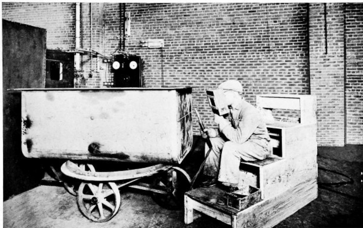
Welding on the end-piece of a tank using a Metallic Electrode.
