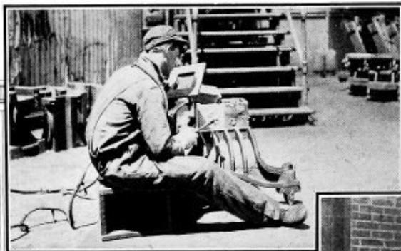
Welding a worn electric railway truck spider.
