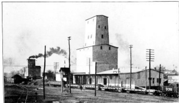
Grain Elevator of John Wade & Sons, Memphis, Tenn., equipped throughout with Weller machinery. The Elevator shown in the background and owned by Davis & Andrews, was also equipped by us.
