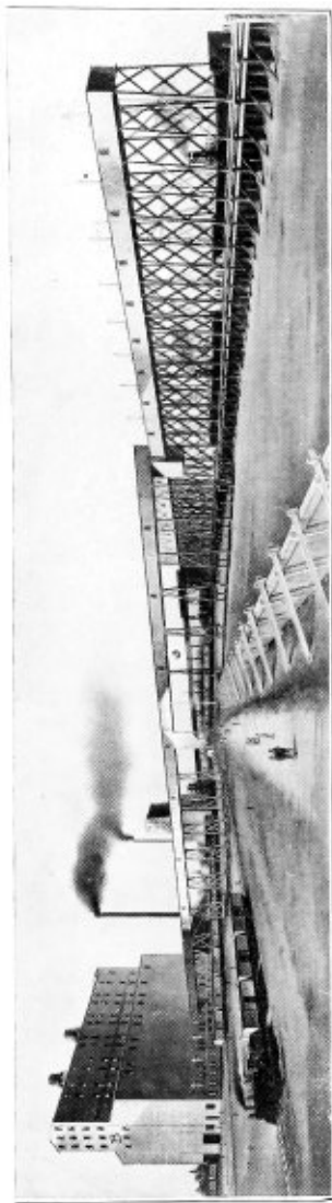
Elevators A and B, of the Texas & Pacific Ry. Co., Westwego, La. The dock conveyors on river front are 1,600 feet long, providing berths for three of the largest ships which can load at the same time. Capacity of Elevator "A," 250,000 bushels; Elevator "B," 1,000,000 bushels. Complete equipment for Elevator "B" and all dock conveyors furnished by us, also machinery for remodelling Elevator "A."
