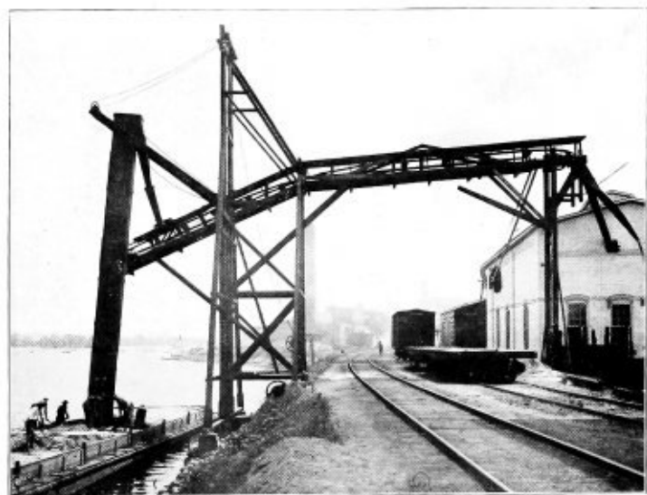
Marine Leg and Belt Conveyor for handling sand, furnished the Tri-City Sandstone Brick Co., Moline, Ill.
