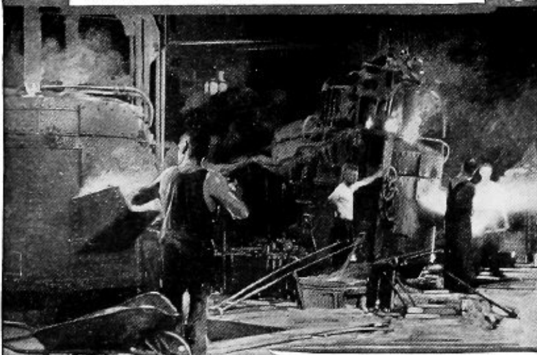
Battery of electric furnaces where electric steel pinions, gears, etc., are made.
