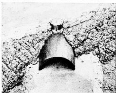
Showing installation of Orangeburg System of Underfloor Duct in a floor of over 3" fill. Note "pad" or "bench" provided under duct and inconspicuous floor outlet.
