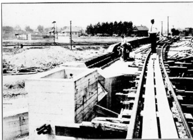
Fibre Conduit incorporated in retaining wall.
