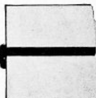
Upper brick placed and tapped down until Johns-Manville Refractory Cement has squeezed out at edge of joint.
