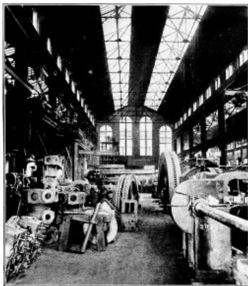
Demands of extremely heavy duty being satisfactorily met by Johns-Manville Industrial Flooring in the shop of the De La Vergne Machine Co., New York.
