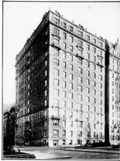
The walls and floors of this structure built by the Horton Building Co. are sound deadened with Johns-Manville Housline. Schwartz & Gross, Architects.
