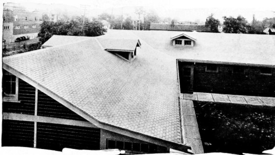
Flexstone Asbestos Shingles afford better service and greater fire protection because of their all-mineral, asbestos rock fibre felt base.
