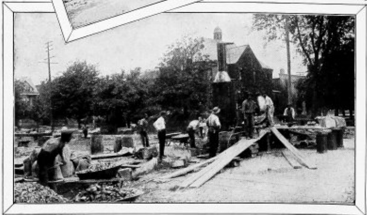
Albany, N. Y. Street Paving
