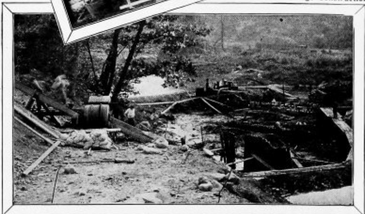
Newburg, N. Y. Bridge Construction
