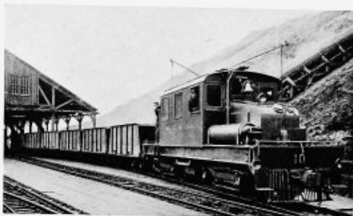
42-ton 4-motor haulage locomotive equipped with air brakes and HL control. This locomotive is used for hauling ore from the mine to the smelter at a Canadian copper mine
