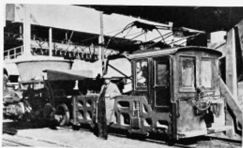
A smelter locomotive, with end cab and air brakes, used in handling slag cars and concentrate at an Arizona copper smelter. Similar locomotives are in service at all large smelters in the West
