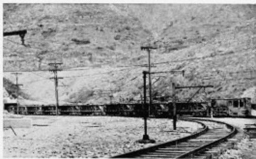
This locomotive hauls ten 25-ton ore cars through a 6600-ft. tunnel to the crushing plant of a large Arizona copper company
