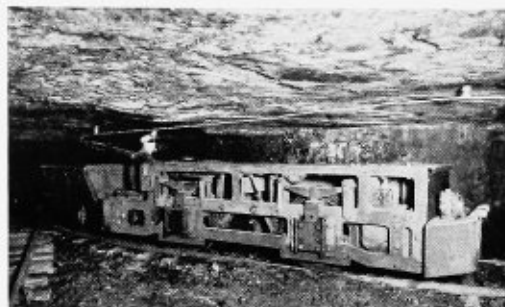
15-ton Barsteel locomotive in a western Kentucky coal mine. The massive construction of this type of locomotive gives strength without sacrificing accessibility
