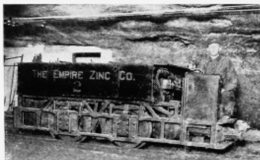
Storage battery locomotive in underground service in a Colorado zinc mine
