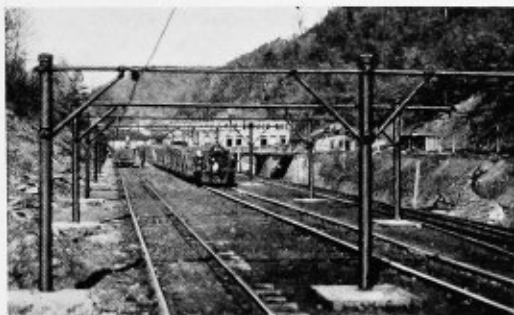
The overhead construction of this Virginia mine is thoroughly modern and consists entirely of Westinghouse equipment
