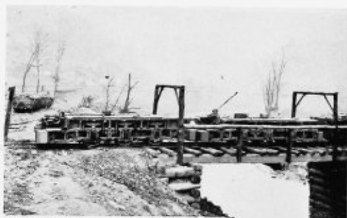
Special tandem unit consisting of two 3-motor locomotives with magnetic control built for a West Virginia coal company to meet the requirement of a heavy locomotive used on narrow gauge
