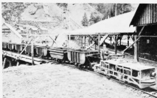
This locomotive operating in a Canadian copper mine is equipped with a special trolley which can follow a trolley wire located on either side of the track
