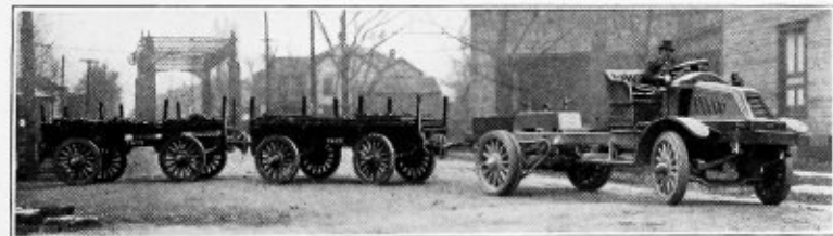
Three Trailers Following Motor Around Right Angle Corner
