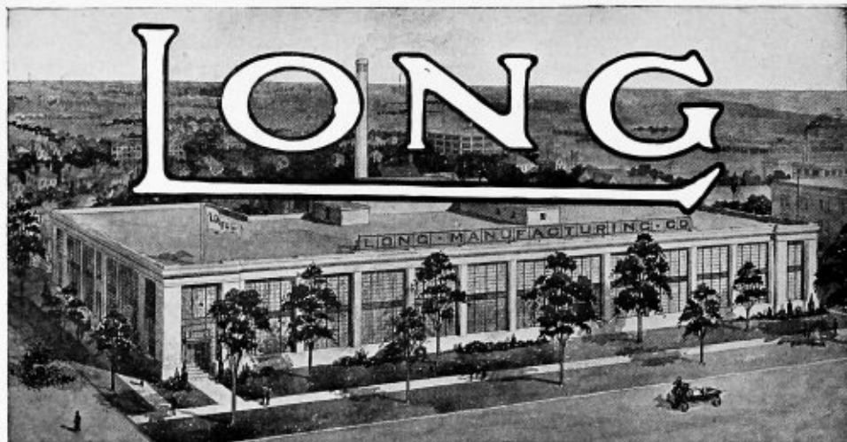
THE MODERN PLANT OF THE LONG MFG. CO., DETROIT, MICH.
