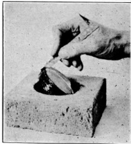
Fig. 3.—Removing Broken Light.
