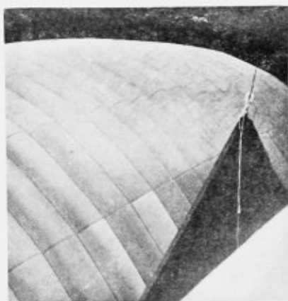
This Pneumatic Roof Was Designed by Paul Poiret, Noted Fashion Creator. The Roof Is Made of Rubber and Can Be Inflated Like an Automobile Tire. In Fine Weather It Is Taken Down but in Rainy Weather Is Immediately Pumped into Place. The Theatre Is Called the Oasis
