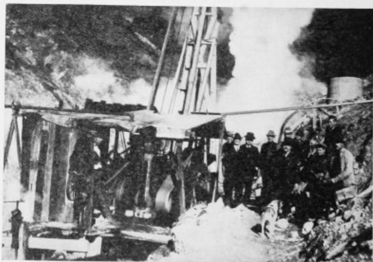
The First Power Taken from a Geyser. The Photograph shows the Steam Engine Developing 1500 Horsepower from Natural Vents in Geyser Canyon
