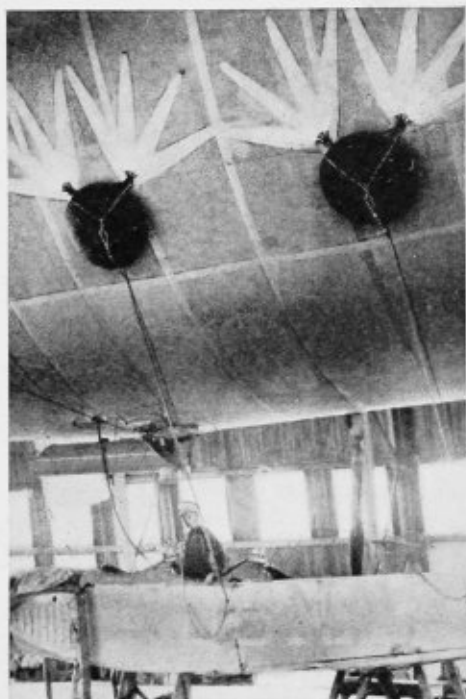
The New Type Parachute Containers Hang on the Side of the Airship Gas Envelope. The Lid Is Supported Only by a Cotton String
