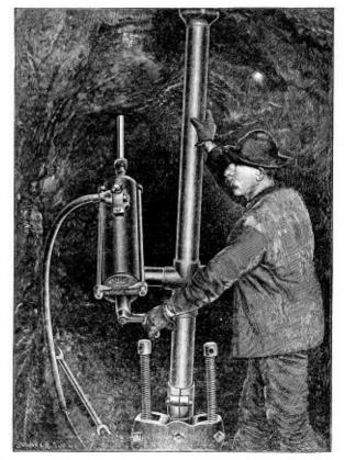
expansed by electric drills. — The air plant was situated 1.000 feet higher up the mountain than was required with the electric drill and the finel had to be carried to the air plant this increased distance over that necessary for the electric percussion drill.
