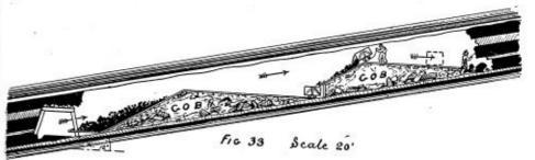
modifications of it, will come much more into use in the future in localities likely to favor its adoption. The leading feature of it lies in substituting or replacing the coal, as taken out, with material put in compact and solid from floor to roof as the work advances.
